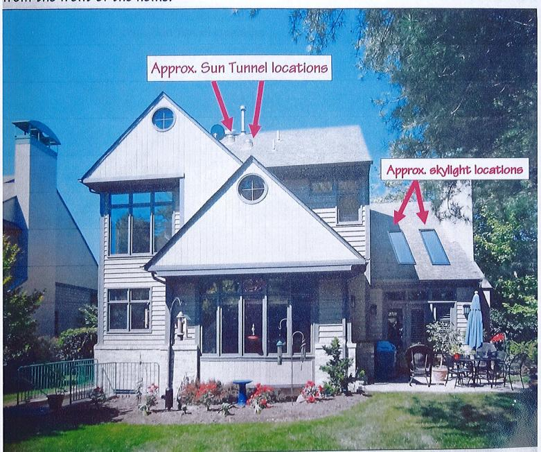
Above photo of the home shows Photoshopped images at approximate intended locations of 1) two Velux CO6 (21.5"x46.25") skylights in roof of the Family Room, and 2) two Velux Sun Tunnels on the rear of the upper level roof above the attic. A close-up view of the locations is shown on next page.
